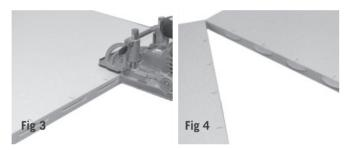
7. Bring the two worktops together and align the front edges and level top surface using either of the two methods below;
