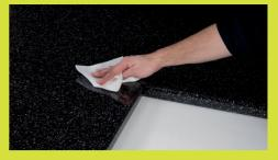
Moisten a clean, lint-free cloth with white spirit and carefully remove the residue, wiping at 90° across the joint to avoid removing adhesive before the joint cures.
